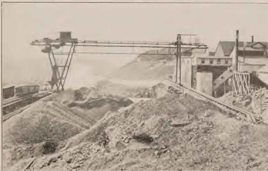
Magpie mine: ore bridge and stock pile.
